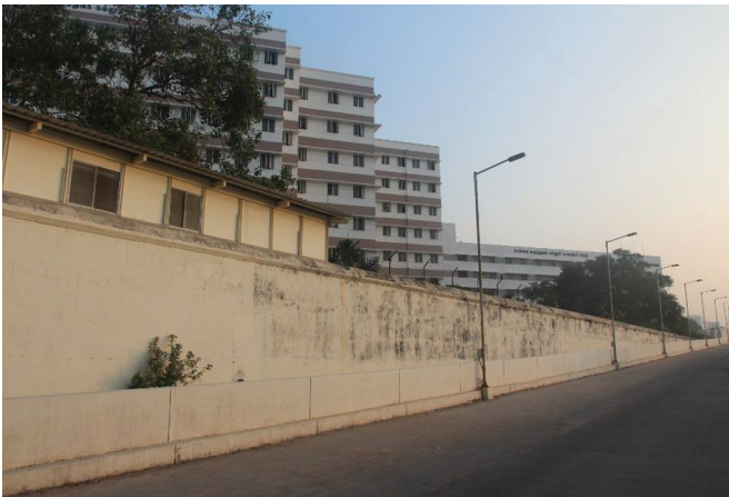
FIG 8. Vestiges of the high-security outer perimeter fence of the central jail in the new medical college premises
