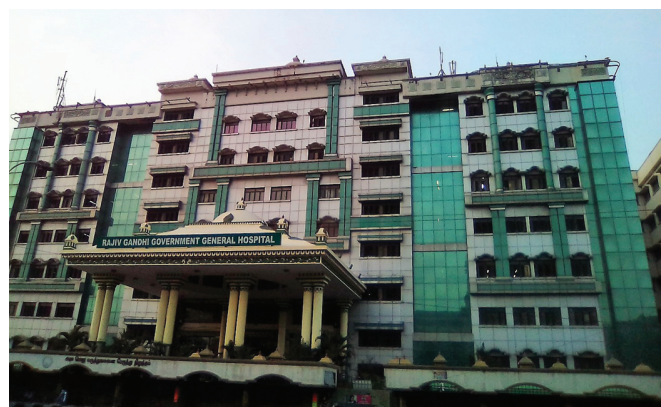
FIG 5. The six-storeyed tower block of Rajiv Gandhi Government General Hospital today
